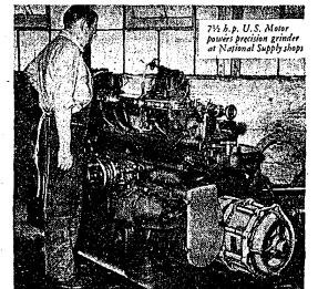
For eighteen years this U. S. Motor has delivered faithful. trouble-free service in the National Supply Company shops. It is shown here powering a Norton Universal Grinder, in a super finish grinding operation. National Supply uses many U.-S. Electrical Motors in the manufacture of its extensive line of high quality oil field equipment.
